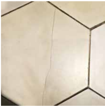
substrate failure
