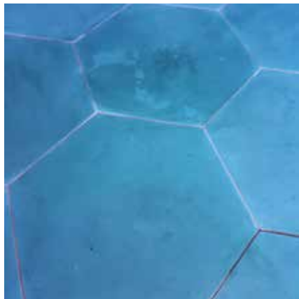
using epoxy grout remover
