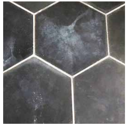
efflorescence
